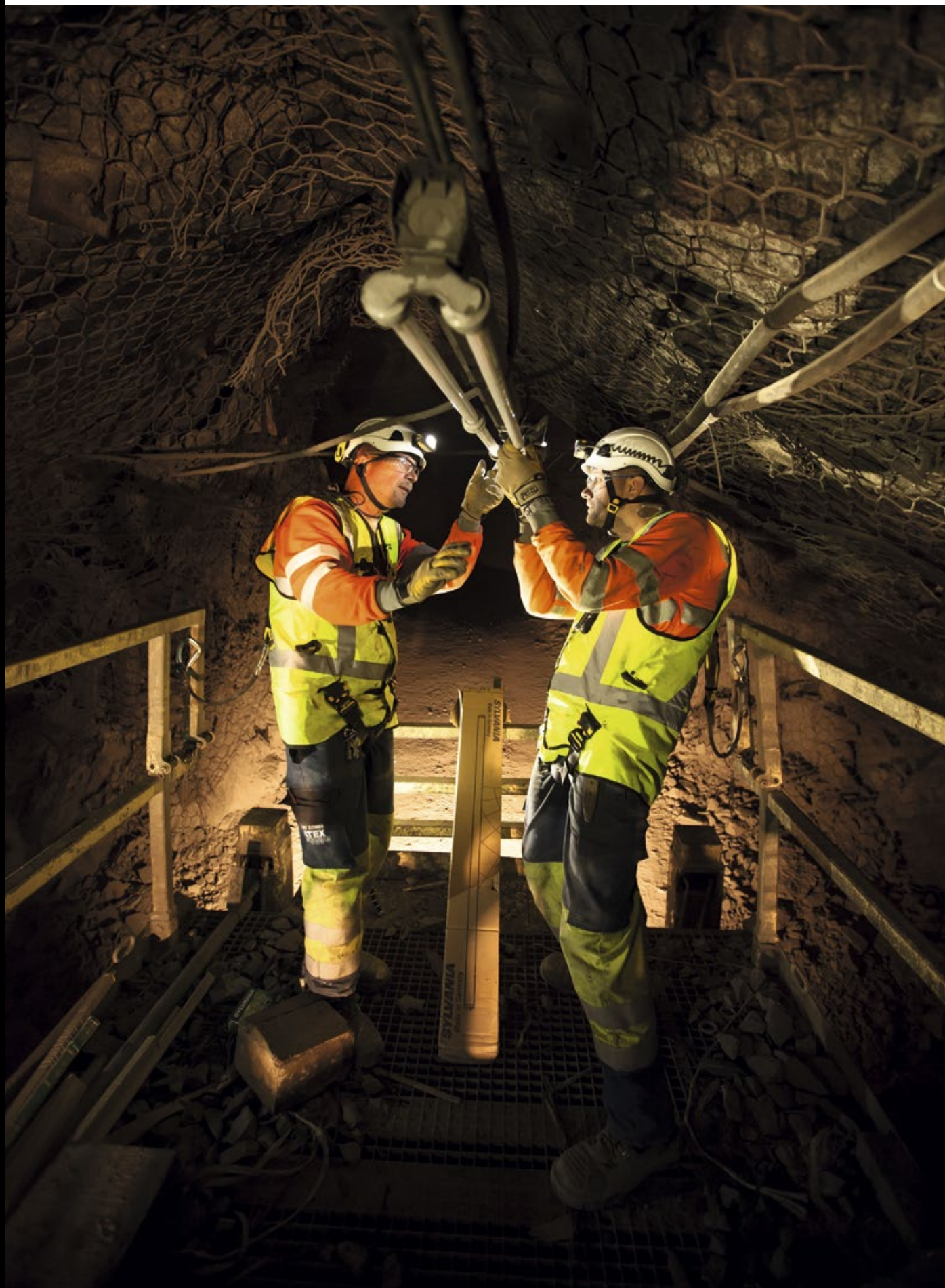
Replacement and maintenance of the lighting system inside a cement mine. © Petzl / Lafouche / Vicat
